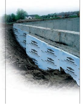
R-value (R-5 per inch) and exceptional moisture resistance. Its proprietary closed-cell structure enables it to defend against all forms of water and water vapor, so it maintains a stable R-value over time.
